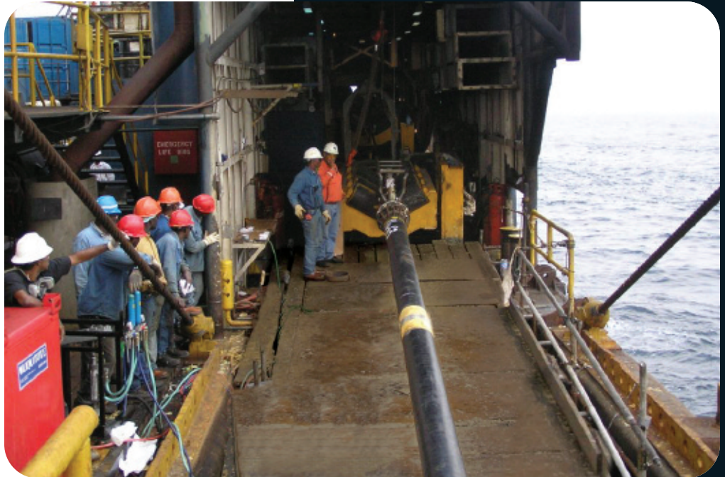
On-site Field Joint Coating System
