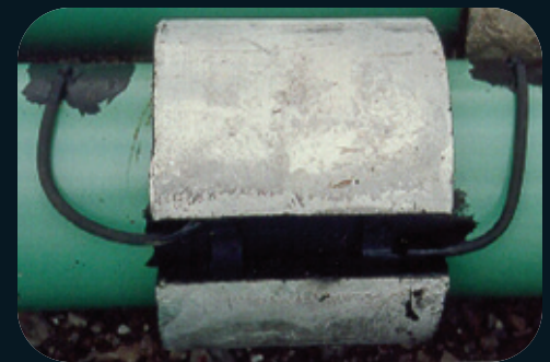
Anode Tapers before FLOMAX FT-6000 elastomer
